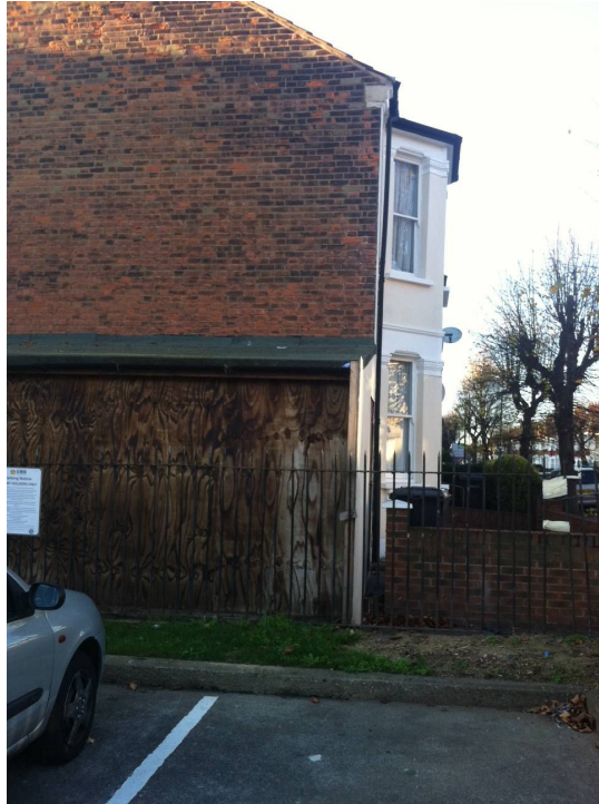
The shed to the side of 1 Dunbar Road
